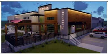
Proposed perspective view of the building shows the change of materials from EIFS to cedar lap siding (wooden), fewer awnings, increased header height along the north wall, increased height of canopy and wall sign and eliminating the projecting sign. Proposed work will also include a covering over the patio area.
